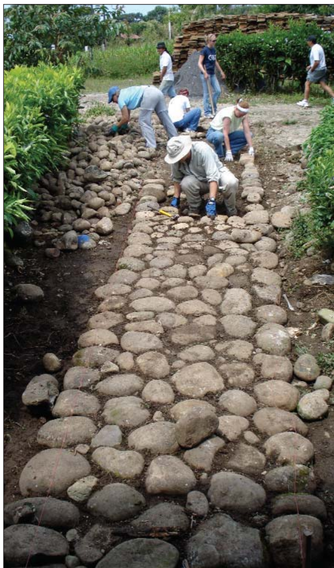
Rebuilding the stone path
